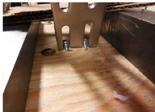
Photo 4: Closeup of Fastener Pullout
