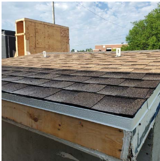
Photo No. 1 Top Side Before Testing
