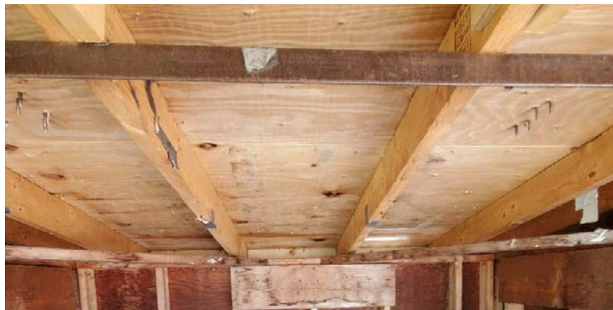
Photo No. 6 70 MPH Underside
