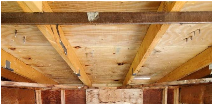
Photo No. 4 35 MPH Underside
