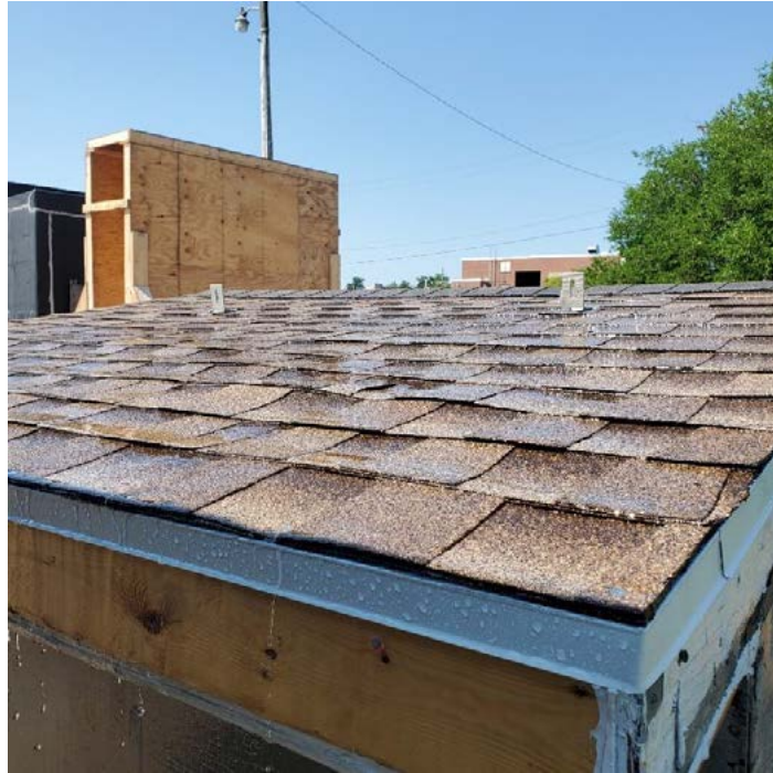
Photo No. 11 Post Test Top Side
