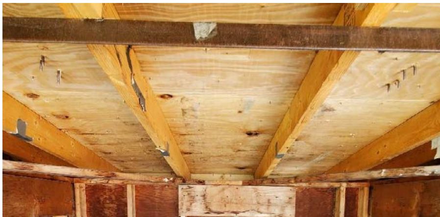
Photo No. 2 Underside Before Testing
