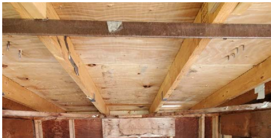
Photo No. 8 90 MPH Underside
