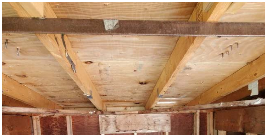
Photo No. 10 110 MPH Underside
