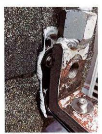
Figure 4c. Bolt failure mode.
